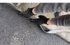
Corabit KK Joint Tape is a cold-adhesive, co-extruded bitumen-based joint tape with a synthetic adhesive layer developed for road construction.
