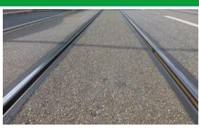
The Corabit ES is elastically adjusted, so that movements are absorbed and flank tensions are well reduced. By using elastomer-modified bitumen, Corabit ES remains flexible even at low temperatures.
