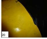
Starting at the bottom, heat the The shrinking process is finished Press on the transition to the shrinkable sleeve in the center in the when the cuff with indicator is tight factory coating, the edge of the circumferential direction with a all over and appears smooth and the sleeve, the overlap of the sleeve blue-yellow flame and shrink it. thermal indicator can no longer be and the weld seam area with a
