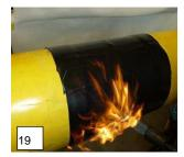
Starting from the center, shrink in felt. the circumferential direction to one side as far as the edge. After completion, start shrinking again from the center in the other direction to the edge.
