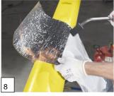
Remove the release film from the beveled end over the entire width and in a length of approx. 300 mm. Heat the adhesive of the sleeve if necessary..
