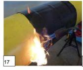
Heat the outside of the closure and press it on.
