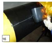
Heat adhesive side further and place over the entire cuff width in the area of the overlap. Work from the inside out with the seam roller to prevent air pockets.
