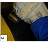
Heat the adhesive side of the closure from one side with the gas flame. Place the heated side centrally on the overlap of the
