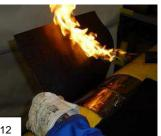
Wrap the shrinkable sleeve thight around the pipe. Align and heat adhesive with blue-yellow flame.
